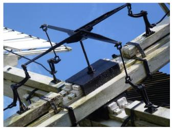
Patent Sails. The vanes are lifted and set from within the windmill, and the amount showing is dependent on the wind speed.
